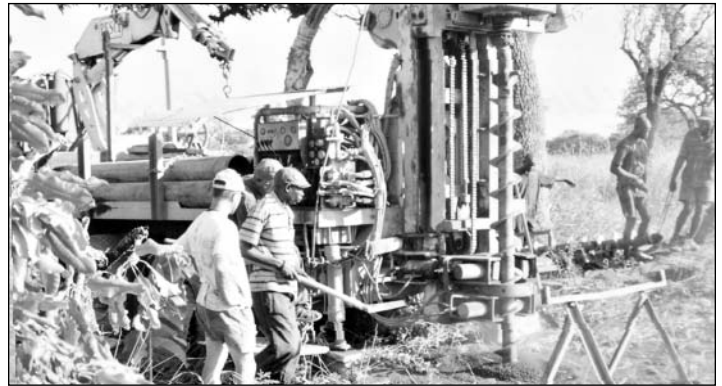
Drilling a well at Archbishop Flynn Secondary School, Feb. 2005
