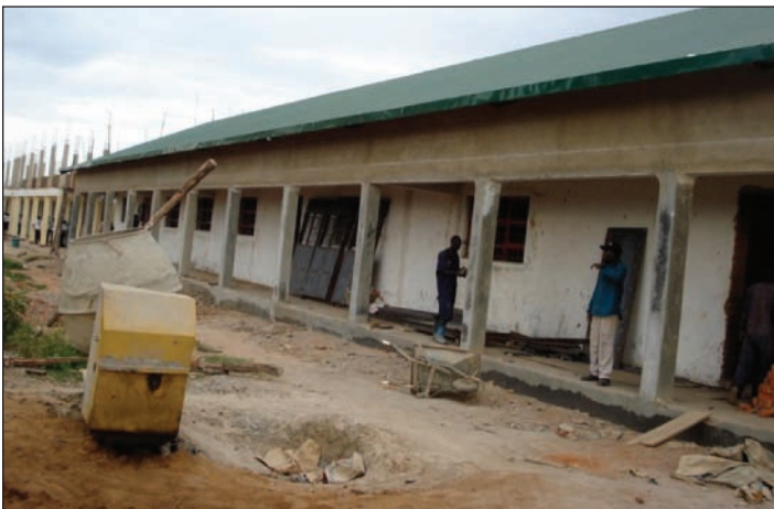
Science Lab nearing completion.
