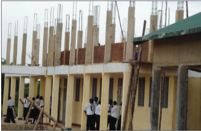
Second Floor of Classroom Block being built.
